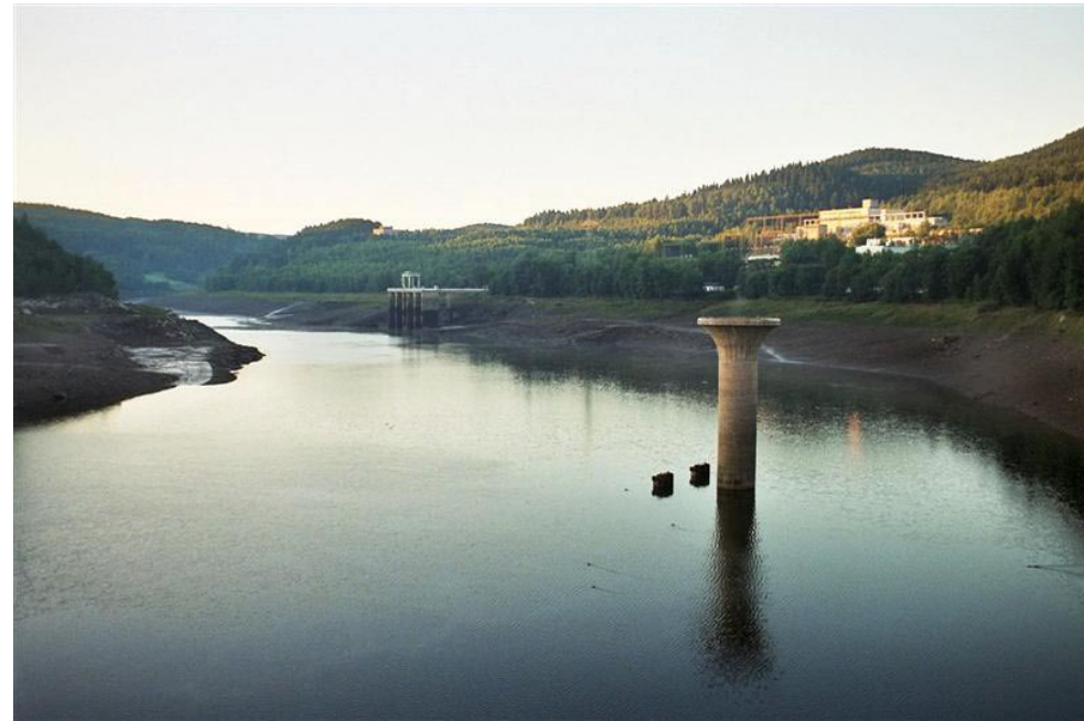
Intake, bell-mouthed spillway, electric utility
